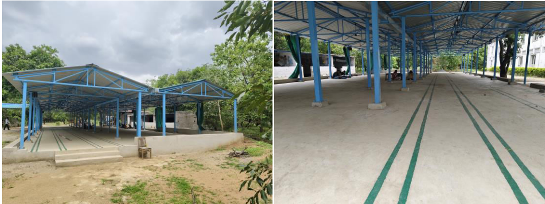
Dining Hall extension at Rollakal School
